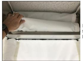
Roll up the top cover and place it in the cove in the header that is located opposite of the ladder.
