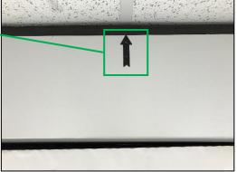
After raising the header close to the ceiling, fine tune the positioning by aligning the arrow marker closest to the back of the unit with the ceiling grid. After adjusting the position as needed, raise the header until it seals against the ceiling. Be sure to lock the casters before entering the unit.
