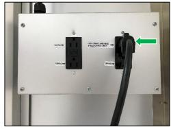
If the PAS750 unit is located inside the AG8000, plug the unit into the outlet labeled "FOR 120VAC VARIABLE SPEED DEVICE ONLY" as shown in the picture above.
